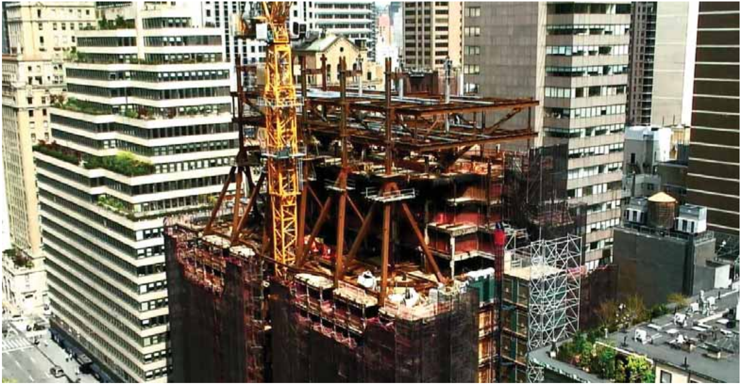
Construction at 425 Park Avenue in May of 2017. Credit: L&L Holding.
