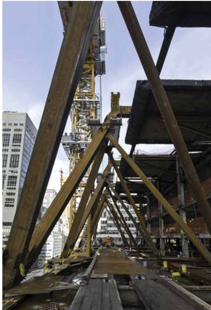
Construction at 425 Park Avenue in May of 2017. Credit: L&L Holding.
