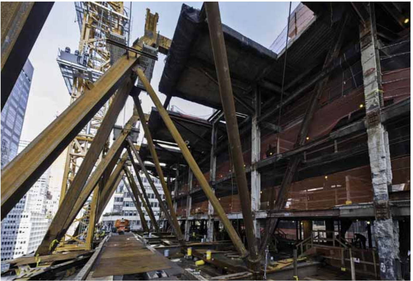
Construction at 425 Park Avenue in May of 2017. Credit: L&L Holding.
